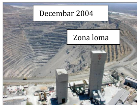
Figure 2 Fracture on the slopes of the open pit in the Palabora copper mine [5]
