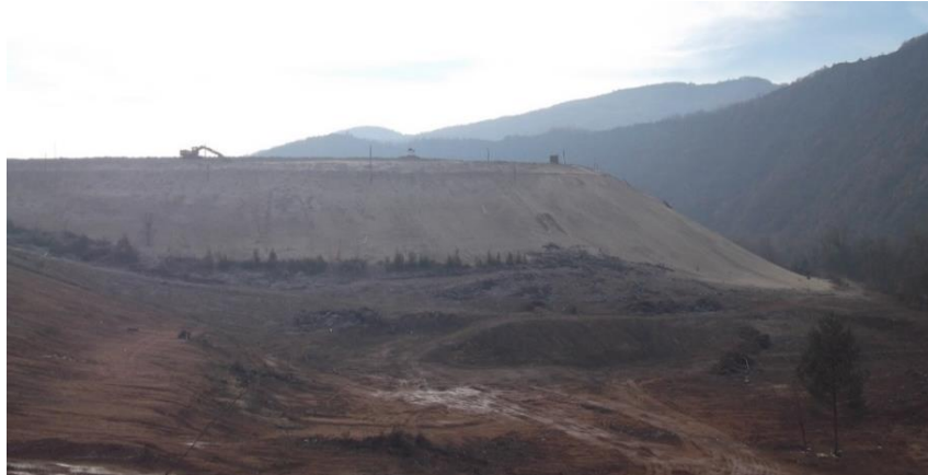
Figure 1 Slope of the Leposavić flotation tailing dump before reclamation
