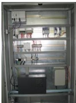
**Figure 7** PLC, I/O modules and equipment for optical communication in Control center
