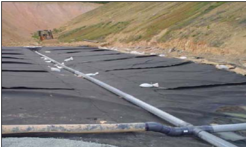
Figure 5. Laying of drainage pipes on the bottom of the landfill
