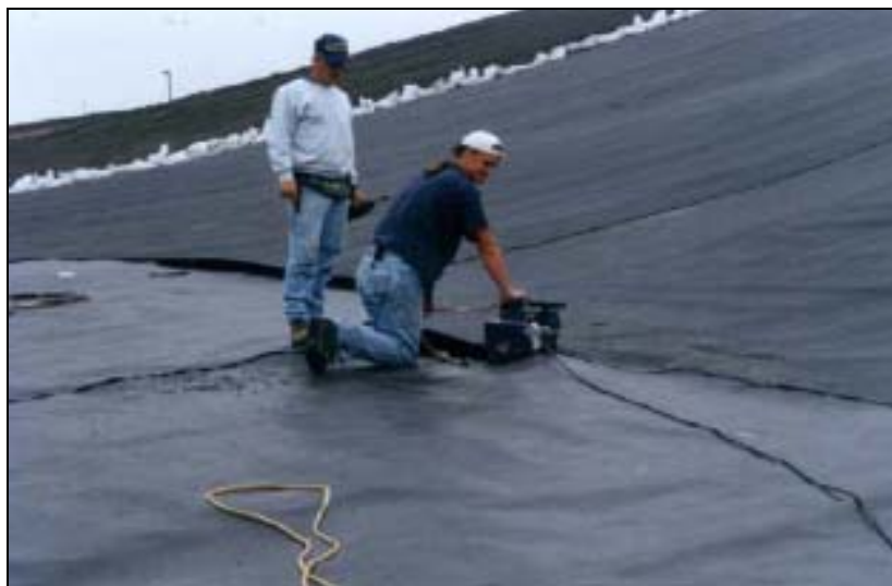
Figure 3. Detail of connecting the HDPE geomembrane
