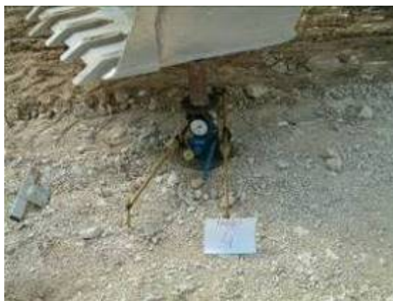
Figure 13. Circular plate at point 4
