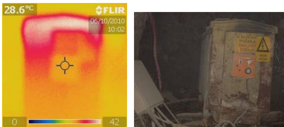
Figure 4. Thermal camera image and standard photo of mine transformer
