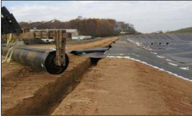
Figure 4. Geomembrane tension by tightening trench and earth
