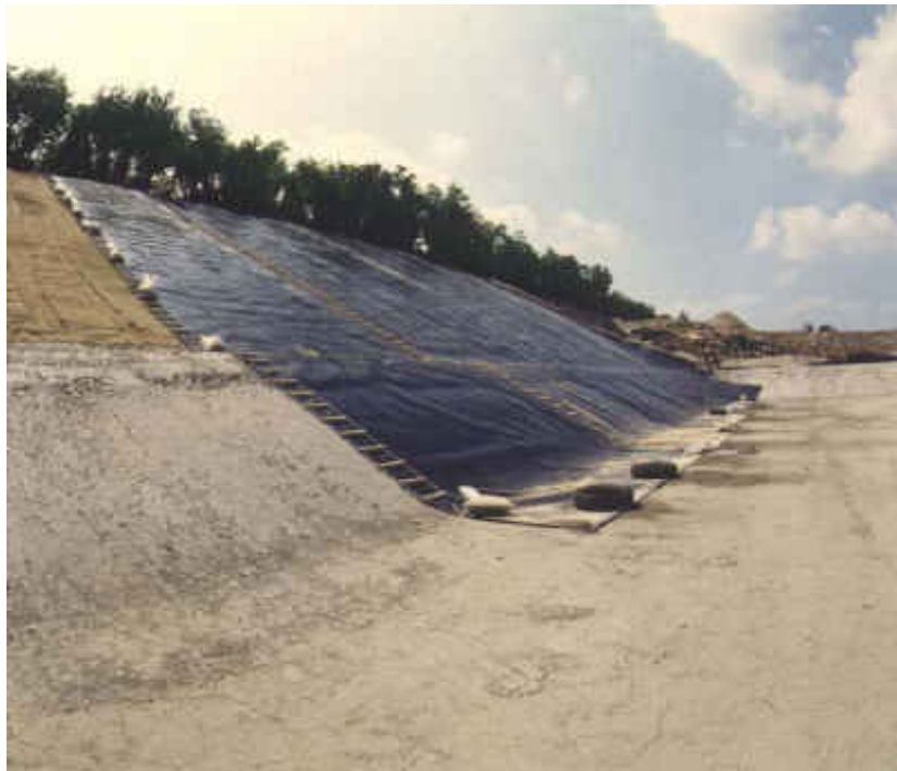
Figure 1. Detail of laying the waterproof film on the inner slope of dam
