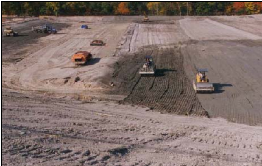
Figure 1. Planning, compacting and flattening the bottom of the landfill
