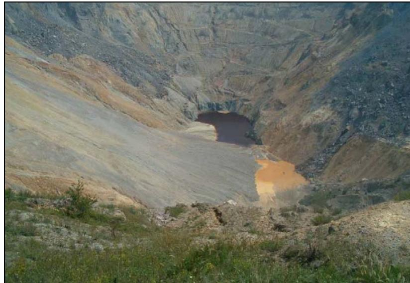
**Fig. 4.** Water accumulation above the ore body Tilva Ros [3]
