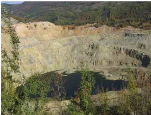
Figure 1. Open Pit Kraku Bugaresku –Cementacija 1 that is expanded
