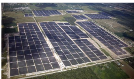
Sl. 11. Sarnia Photovoltaic Power Plant
